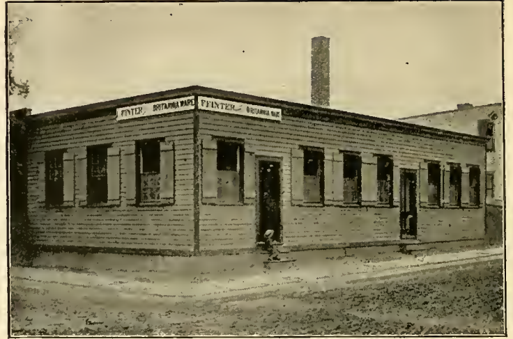
WORKS OF FREDRICK FINTER, CORNER THOMAS AND GOBLE STREETS.
